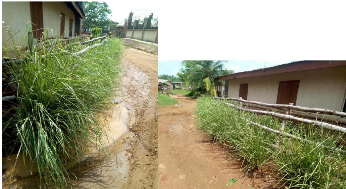
Plate 2 above: shows a house at Eke- Ukwu being protected from erosion using Vetiver grasses
